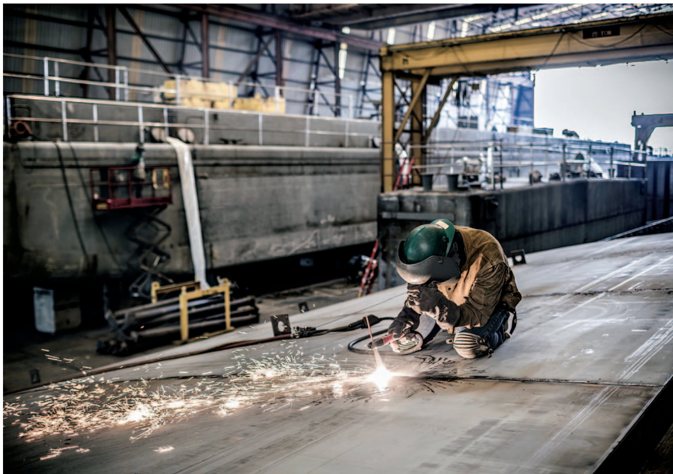
Arcosa Wind Towers worker assembling blade. Photo courtesy Arcosa.
